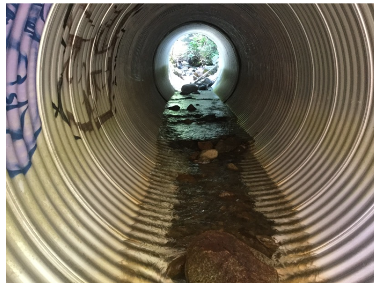
Looking through culvert from outlet
